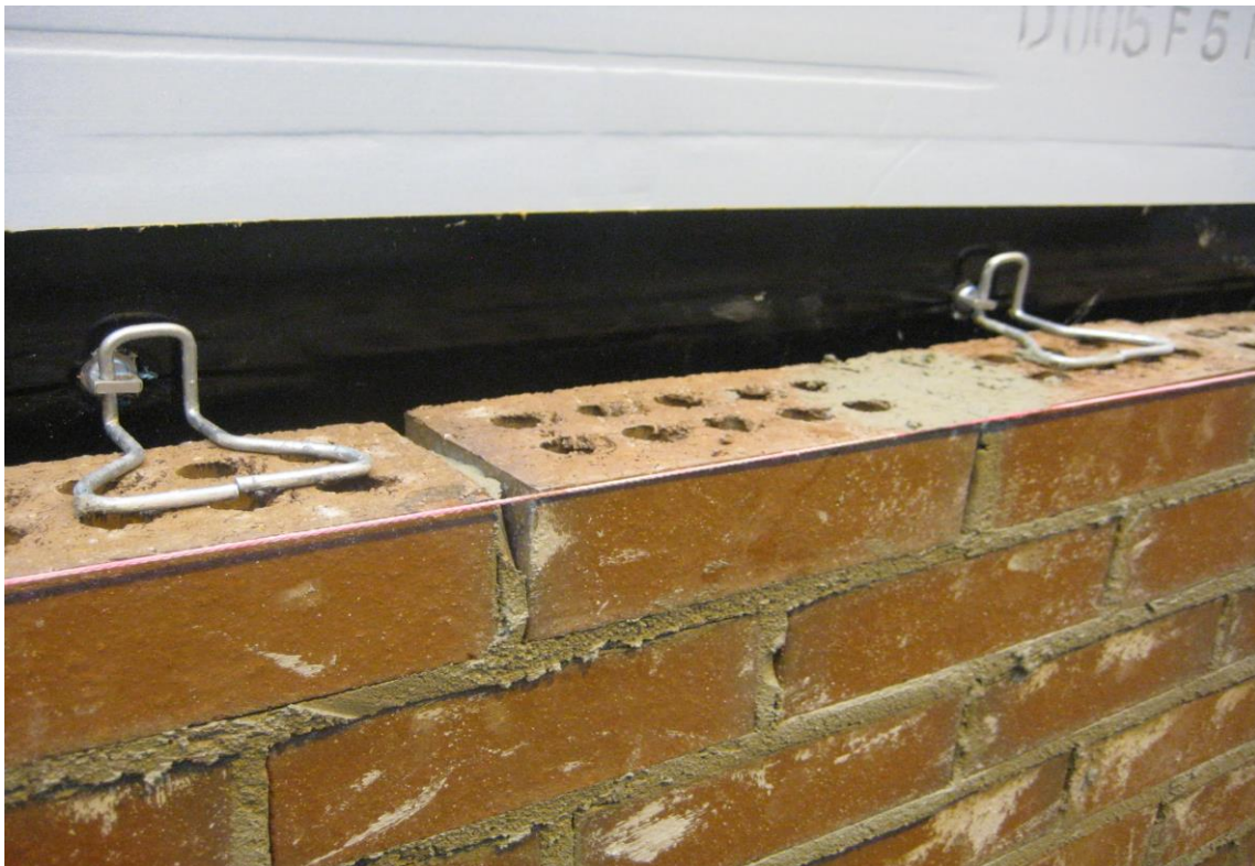
(Exterior of Base Wall, Bricks & Brick Ties being Installed)
