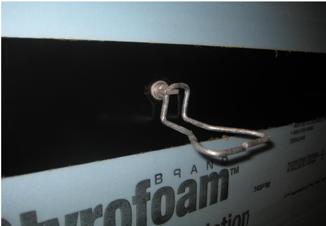
(Brick Tie installed)
