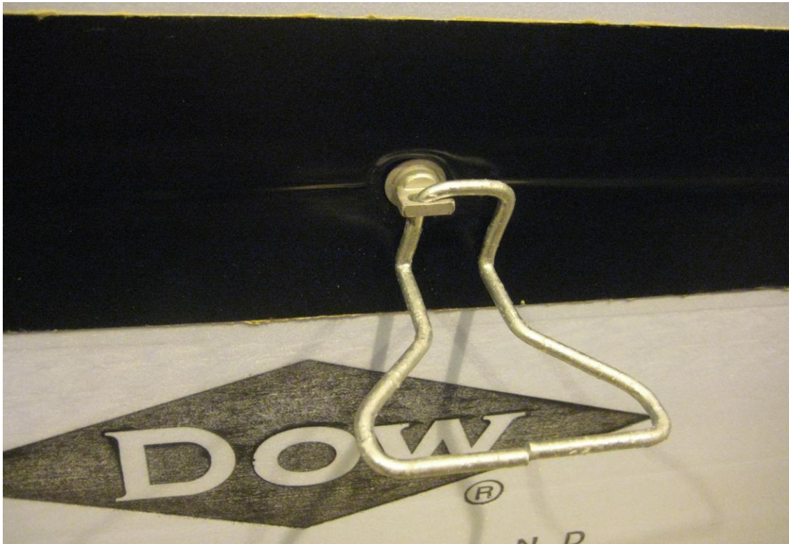
(Brick Tie installed)
